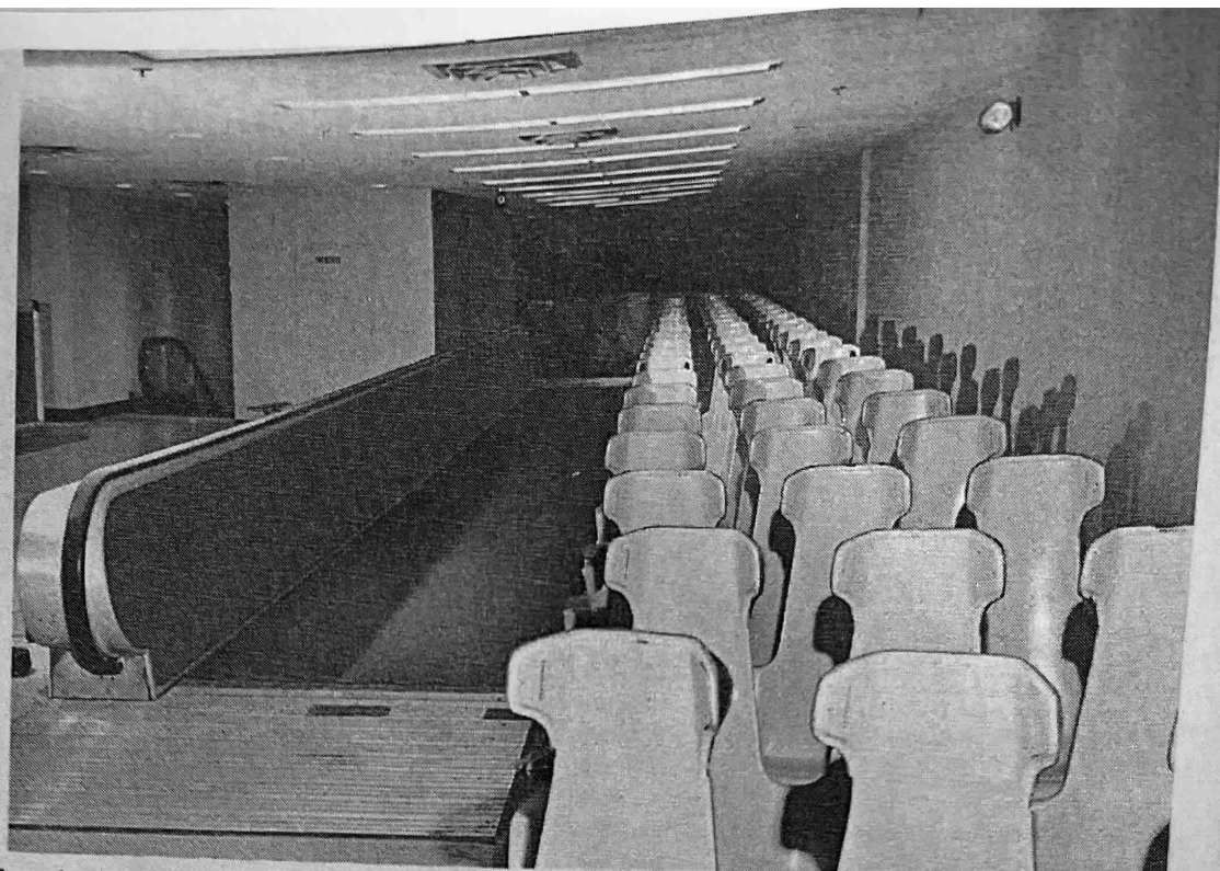
Fig. 10 — Loading and unloading of passengers is accomplished by two moving belt walkways running parallel to the track and moving at the same speed as the ride. One of the walkways is shown here.
